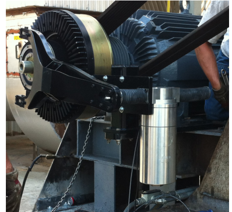
Flux Drive Adjustable Speed Drive (ASD-BP) and Automatic Actuator during installation.
